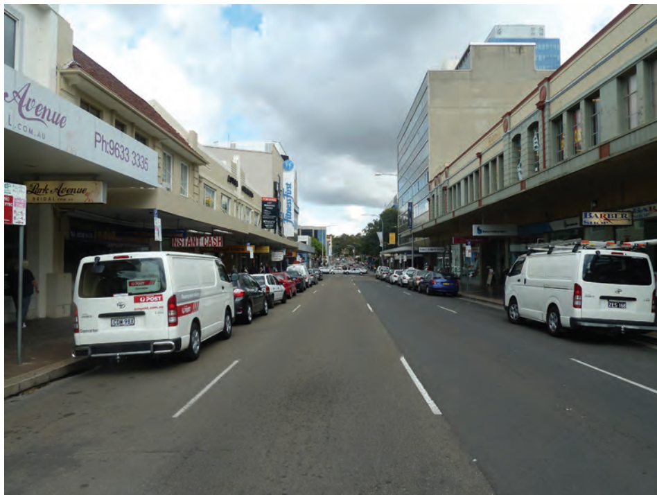
VIEW 13 LOOKING WEST ALONG MACQUARIE STREET
